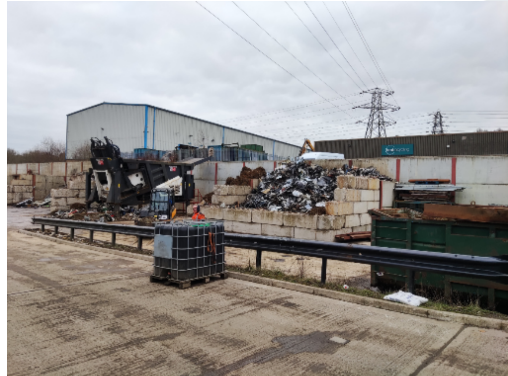
View of south boundary
