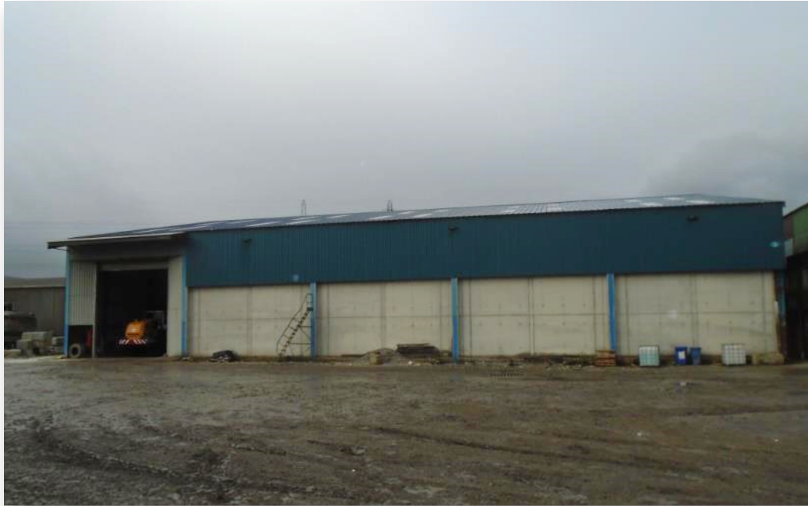
Building B in front of application site
