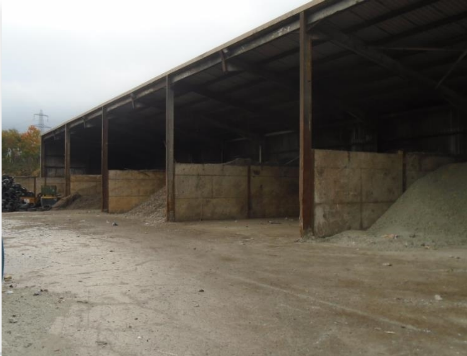
Existing building to be demolished
