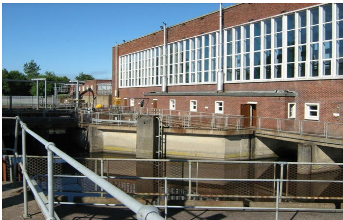
(Crossens Pumping Station inlets)
