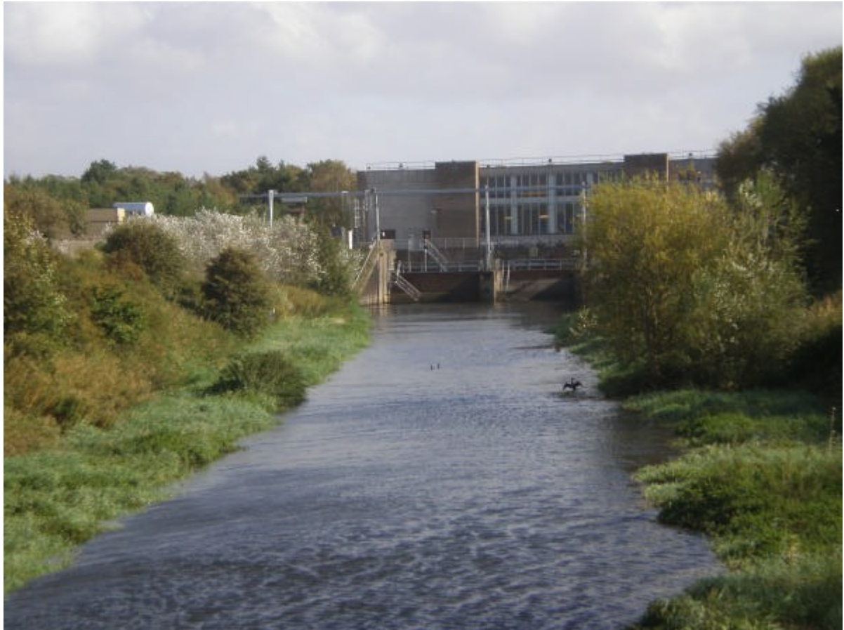
(Altmouth Pumping Station from upstream)
