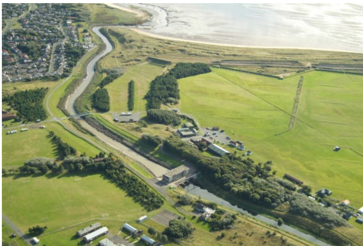
(Altmouth Pumping Station and River Alt Estuary)
