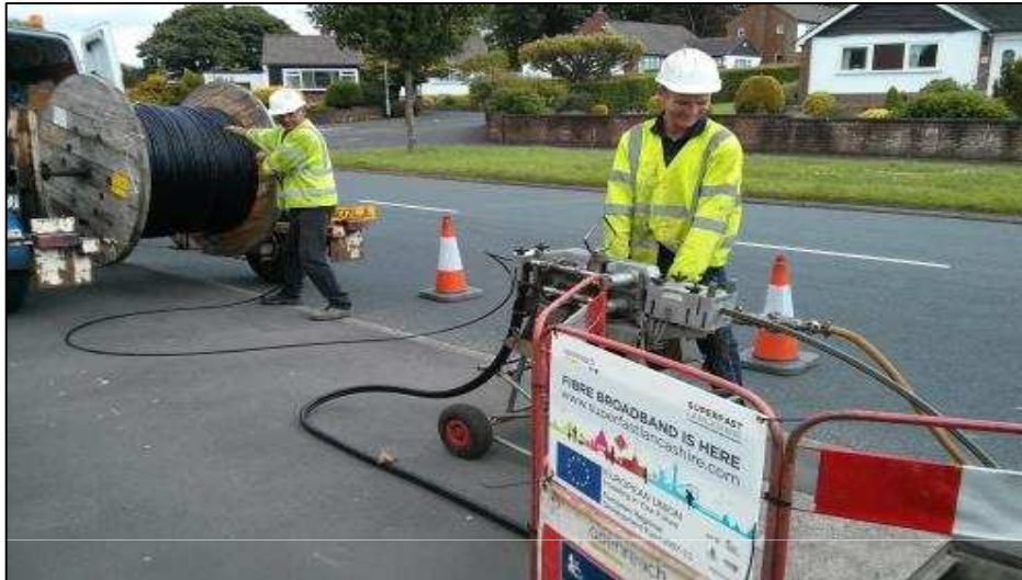
Fibre spine cable being laid between Clitheroe & Chatburn exchanges
