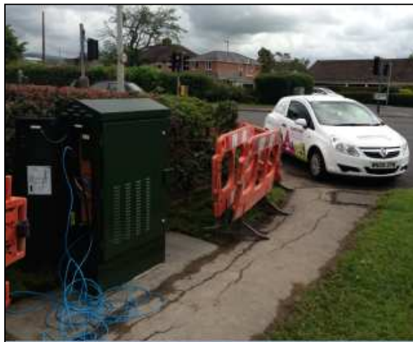
Fibre spine cable being laid between Clitheroe & Chatburn exchanges
