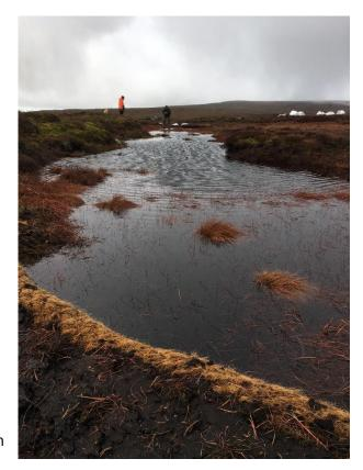
with geo-textile matting to prevent peat loss and installing timber dams and coir logs to reduce water flow off the fell in high rainfall events.
