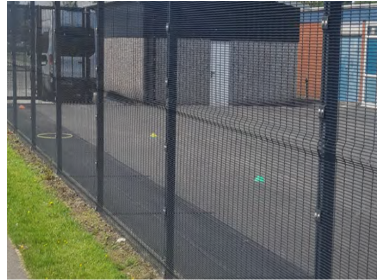
Green Weld Mesh replacement Fencing and Gates
