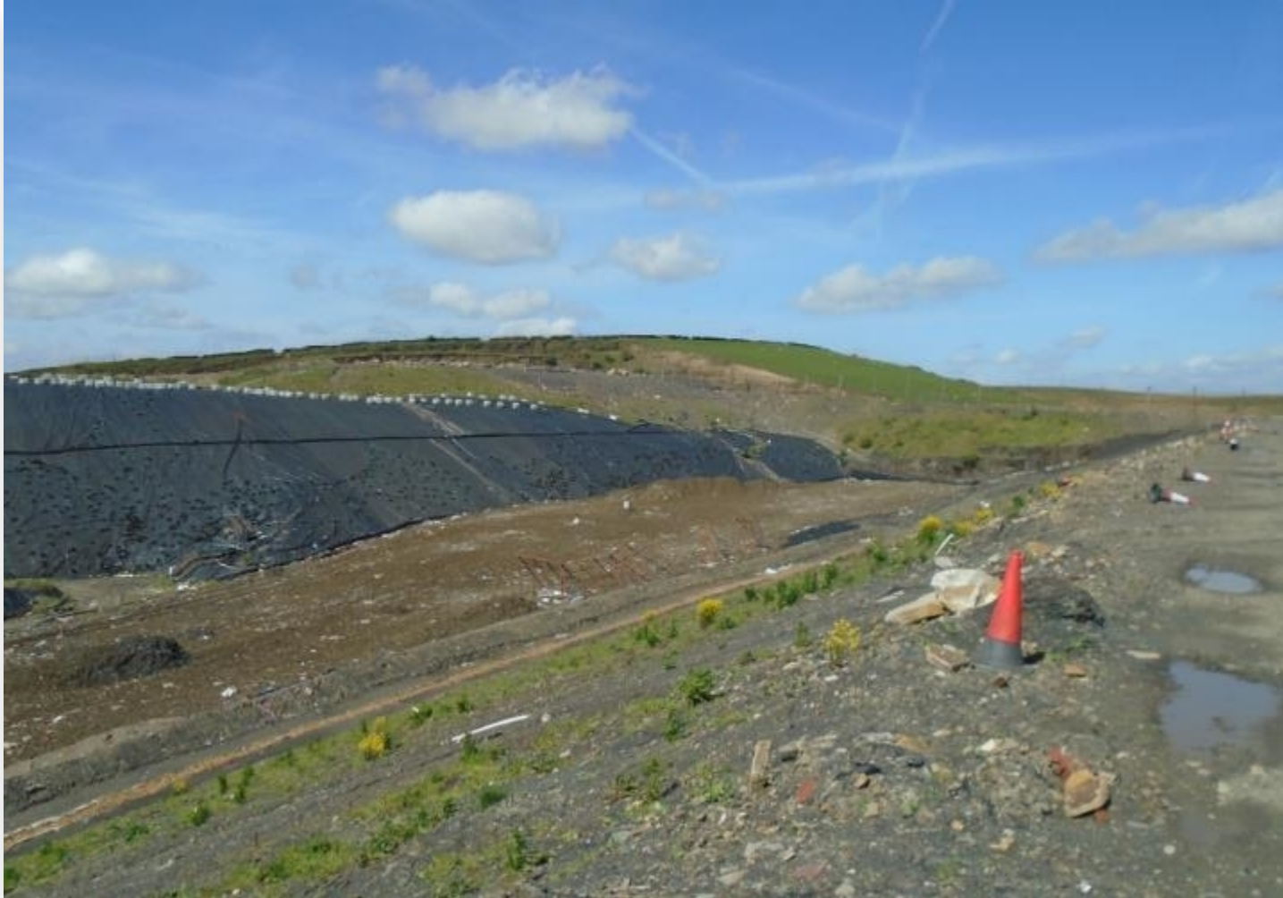
Remaining void space
