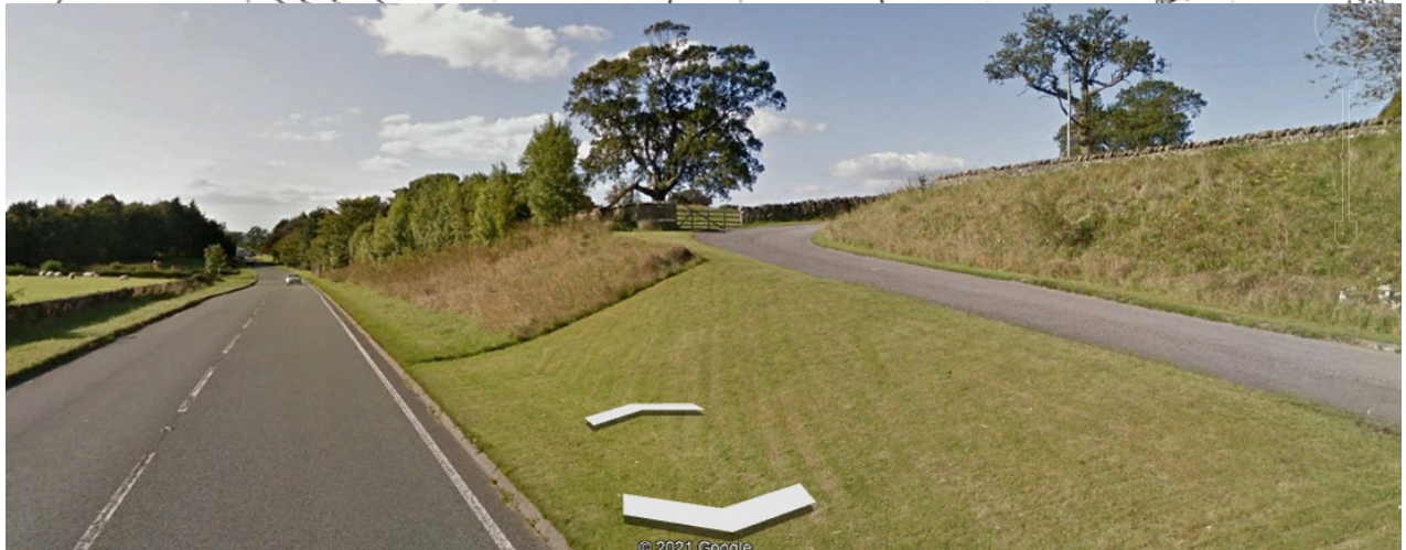
2015 Google Street View of A65 showing steepness of banking
