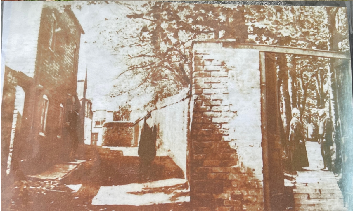
Undated photograph of route under investigation on display on notice board looking back up the route from point C [above]
